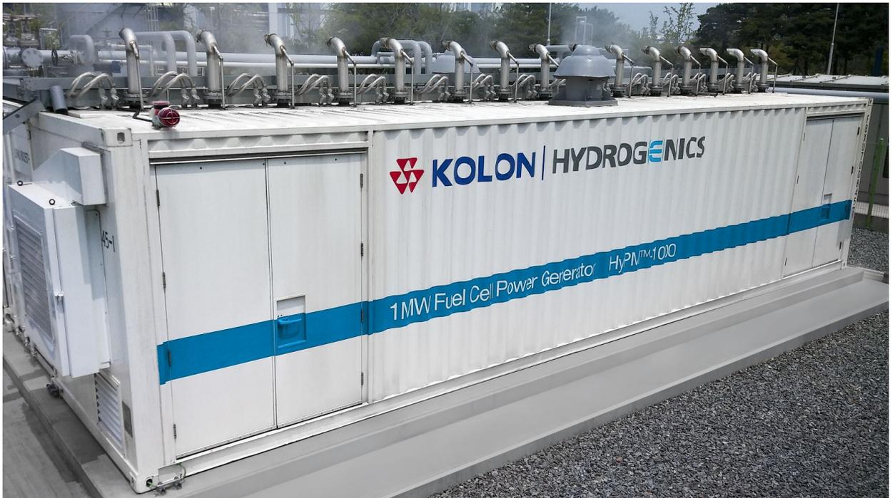
Image 3: Hydrogenics Fuel Cell Megawatt Power Generation
